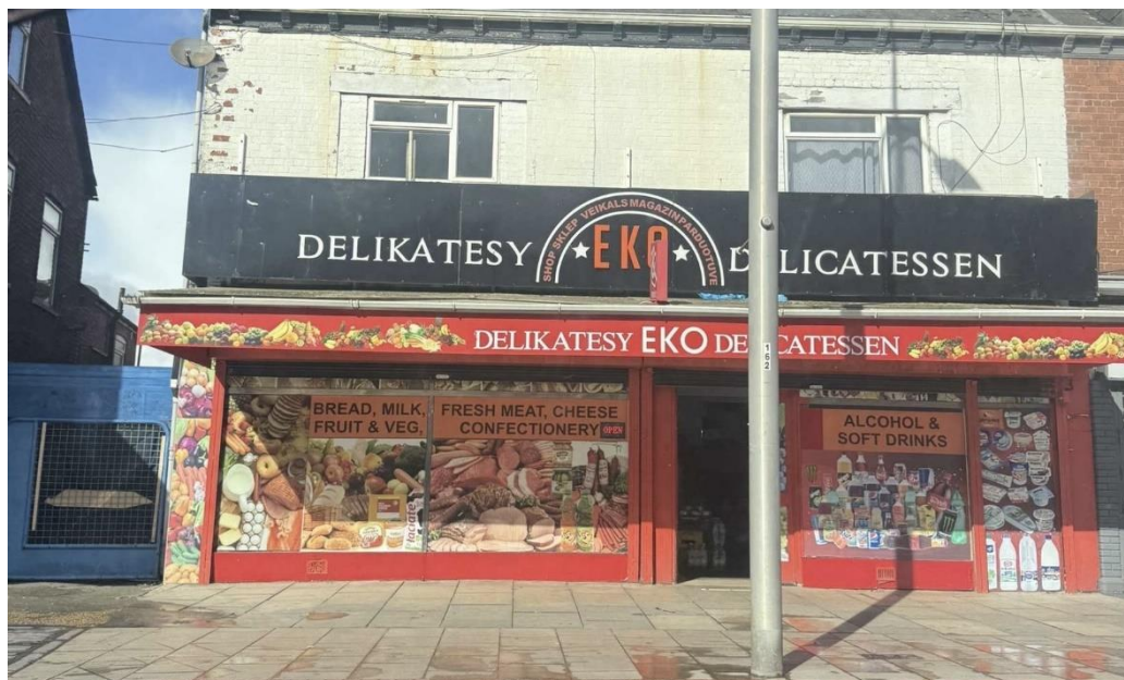
Figure 5.7: Polish Shop on Hessle Road (Author Own, 2025).
